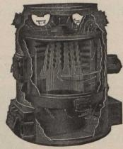
The KELSEY system provides for the constant removal of all exhaled air, replacing it with large volumes of fresh, pure, properly warmed air, ensuring an equable, healthy atmosphere, neither super-heated, nor
