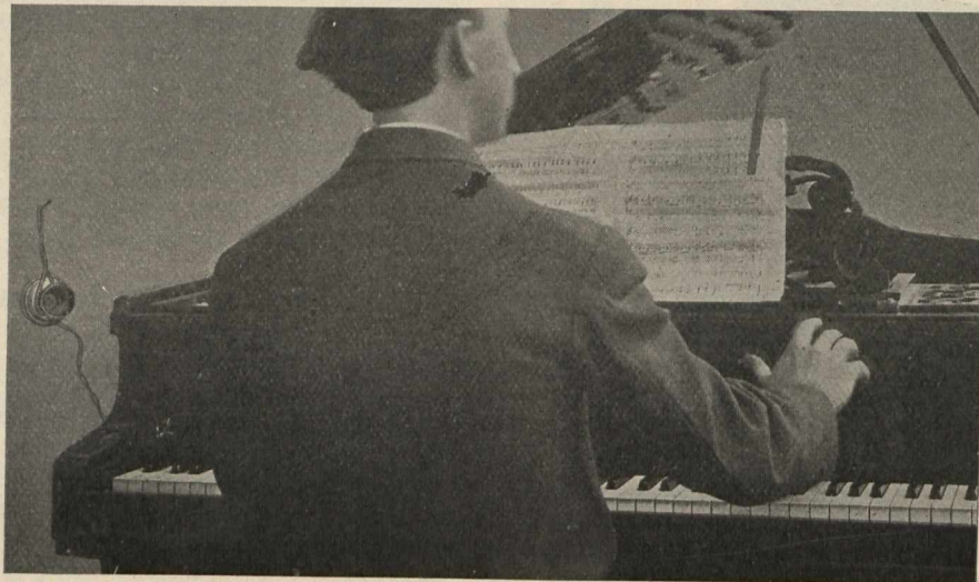
Fig. 2.—Simple Arrangement of Transmitter Suspended on Wall for Transmitting Piano Music.
