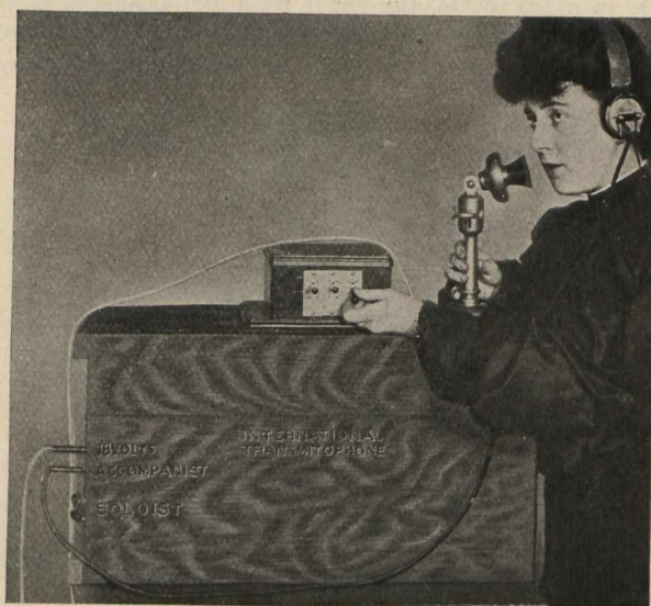
Fig. 4.—One of the Sending Stations Showing Head Receiver Used by Soloist to Assist Her in Keeping Time With Accompaniment.
