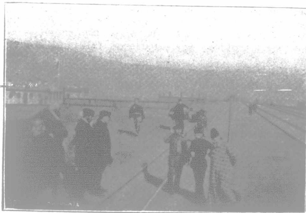
Station in Manchuria.
