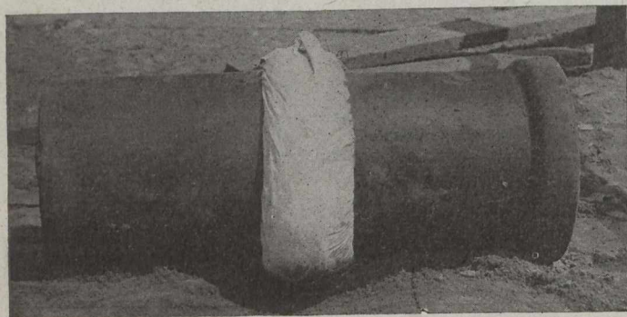
Fig. 2.—Completed Canvas Cover on Joint.
