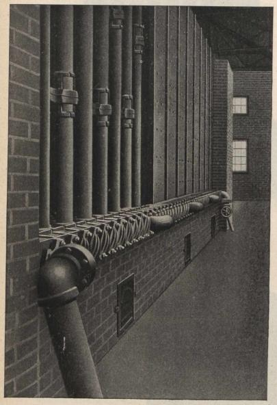
cases where the feed water contains foreign substances, the owners have found these machines to be especially valuable owing to their accessibility and ease of cleaning. An illustrated catalogue describing the Sturtevant "Standard" and "Pony" economizers is issued by the B. F. Sturtevant Co., Hyde Park, Mass., and is of interest to all steam users.
