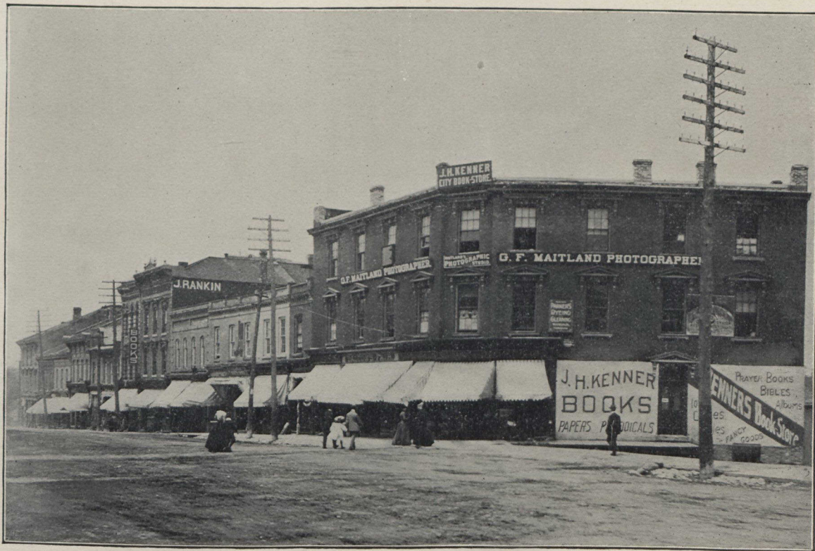
WESTERLY VIEW DOWN ONTARIO STREET
