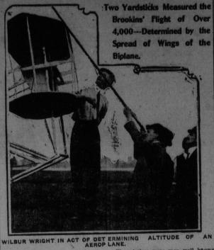
lidianapolis, July 13.—The Wright brothers have a novel and ingenious method of determining the altitude of a Wright biplane. The instrument is as simple as it is ingenious, consisting of a little bit of tin with little projecting spikes or probgs, and a common yardstick, such as department stores give away as advertisements. The tin is bent about the yardstick so that it slips easily from end to end.
