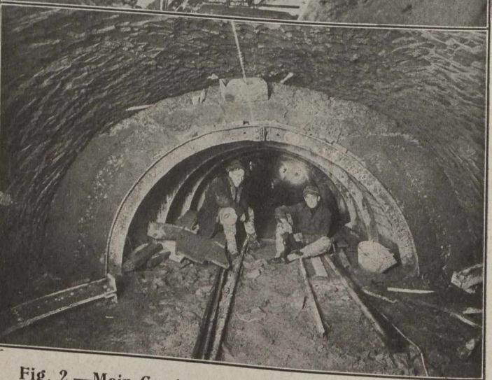
Fig. 4.—Showing Method of Excavating in Tunnel, also Steel Circular Ribs and Lagging in Place. Section No. 4.
