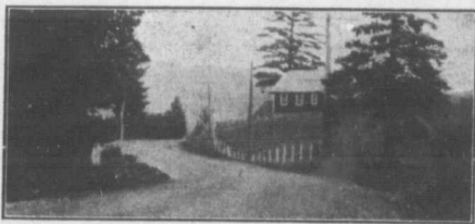
Sherbrooke-Derby Line Highway, Que. Constructed with "Tarvia-X" over slag in 1915.
