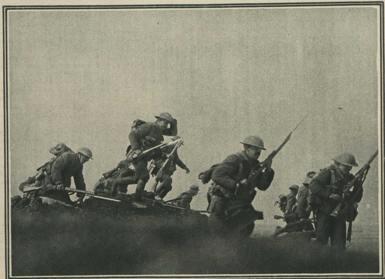
THE MEN GOING OVER THE TOP OF THE TRENCH
