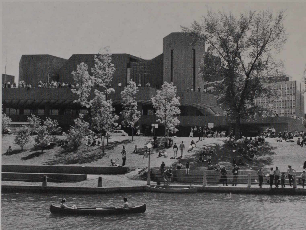
Canada's National Arts Centre on the banks of the Rideau Canal in Ottawa.
