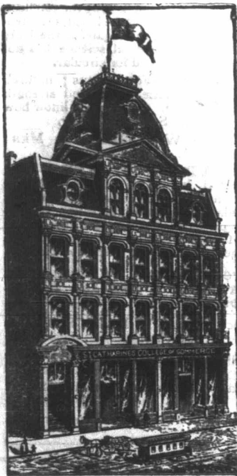
THE COLLEGE occupies the ground floor and first story of this superb structure. It is unquestionably the finest, most thoroughly modern school of business and shorthand training in Canada, and also the cheapest. Circulars free.
