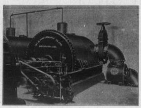
Pair of 35" Special Crocker Turbines one of two pair direct connected to Generators at Station of Sherbrooke Power, Light and Heat Co.
