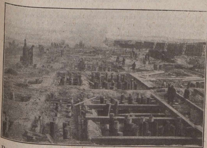
BEARING PILES FOR CONCRETE FOUNDATIONS UNDER ELECTRIC FURNACES IN MELTING HOUSE
