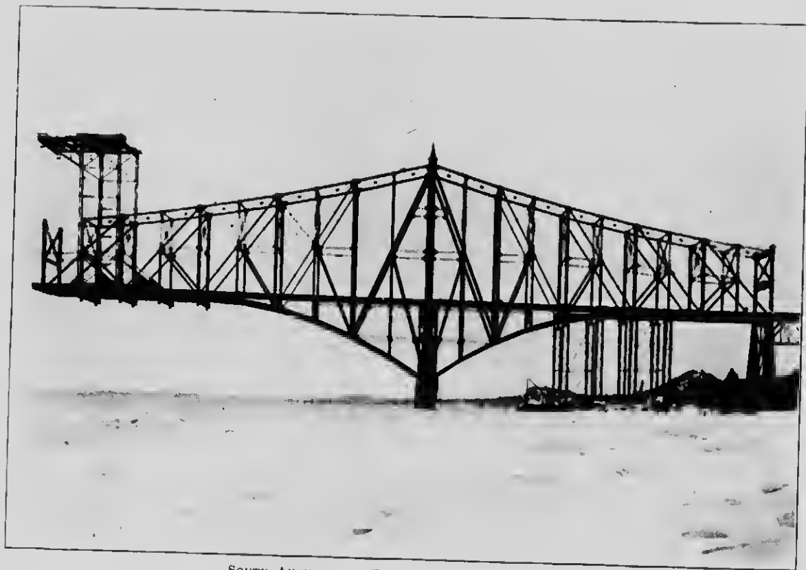
SOUTH ANCHOR AND CANTILEVER ARMS COMPLETE.
