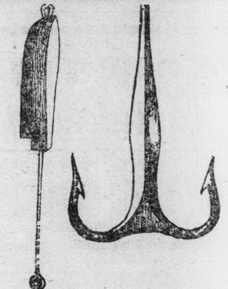
This cut represents the Norwegian Jigger, which is one of the greatest fish killers in the world, and used exclusively in Norway. Can be had from all the Hardware Store in St. John's. Remember it is important to use two swivels in order to make the Jigger spin.
