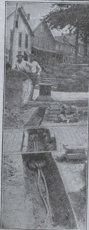
Laying STANDARD Steel-Tape-Armored Cable Across a Street.
