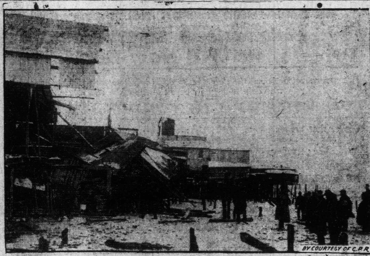
Part of Rockaway Beach, N.Y., after the great storm which smashed four hotels and several iron piers, doing about $2,000,000 damage.
