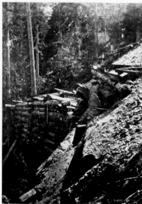
Ore Dump, No. 3 Tunnel, Eva Mine.
