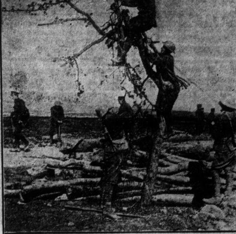
EMERGENCY TELEPHONE POST. The Canadian Engineers across the waters sometimes have to use just an old wreck of a tree for their telephone posts, as in the case of the emergency post seen in the picture.
