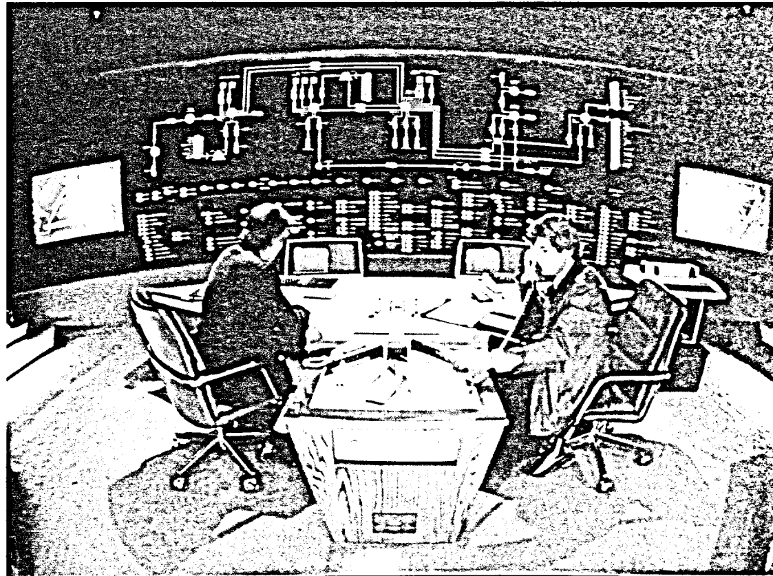
The network control centre keeps an eye on telecommunications traffic to minimize congestion on the international routes.
