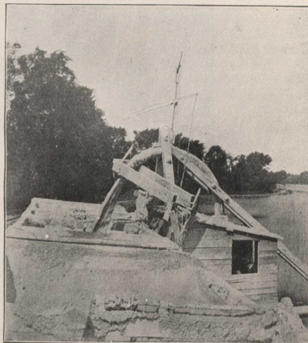
PNEUMATIC SYSTEM OF PUMPING MARL.
