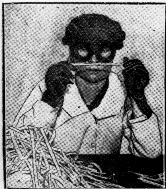
Testing the "bang" part of a Christmas cracker to make sure that it will go off. Scene in an English factory.
