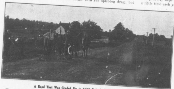
A Road That Was Graded Up in 1909 Entirely With the Split-log Drag The possibilities of the split-log drag are well illustrated in the photo reproduced above. This road in the township of Clinton, near Beamsville, Ont., was turpiked up from the flat by means of a split-log drag.
