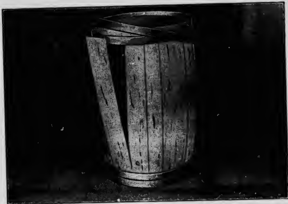
FIG. 1. Stake removed for inspection.
