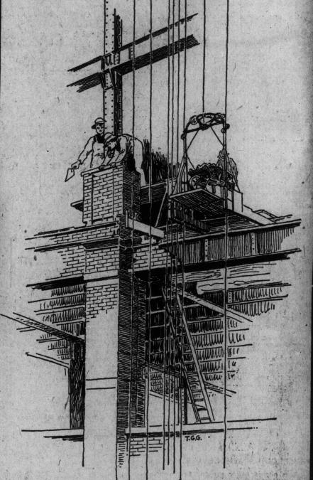
Knox Church. The steel work for this stucture was all made in Canada and not three pieces in the whole outfit failed to fit true in their positions when placed. The columns are supported on cement footings which go down about forty feet below the street level into solid, lead-like blue clay. This building is said to be the biggest block of steel construction in the British Empire.
