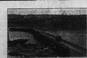
BUFFALO RIVER BRIDGE, CAPE COLONY. All Woodwork, including Submerged Piles, treated with SOLIGNUM.
