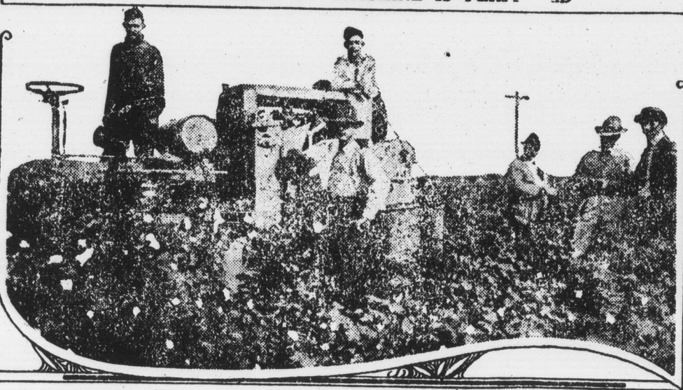
It looks as though science had at last developed a machine that would displace human hands in the cotton field. The machine above is the development of a cotton-picking device invented 20 years ago by Angus Campbell, a Scotchman, and is being used successfully, picking 1200 pounds of cotton an hour, which equals the work of 60 men. It has cost about one million dollars to develop the apparatus to its present state of perfection.
