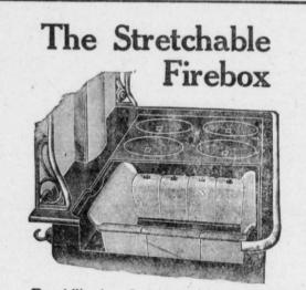
Durability in a firebox depends mostly upon its ability to expand when hot and to contract when cold, without cracking.
