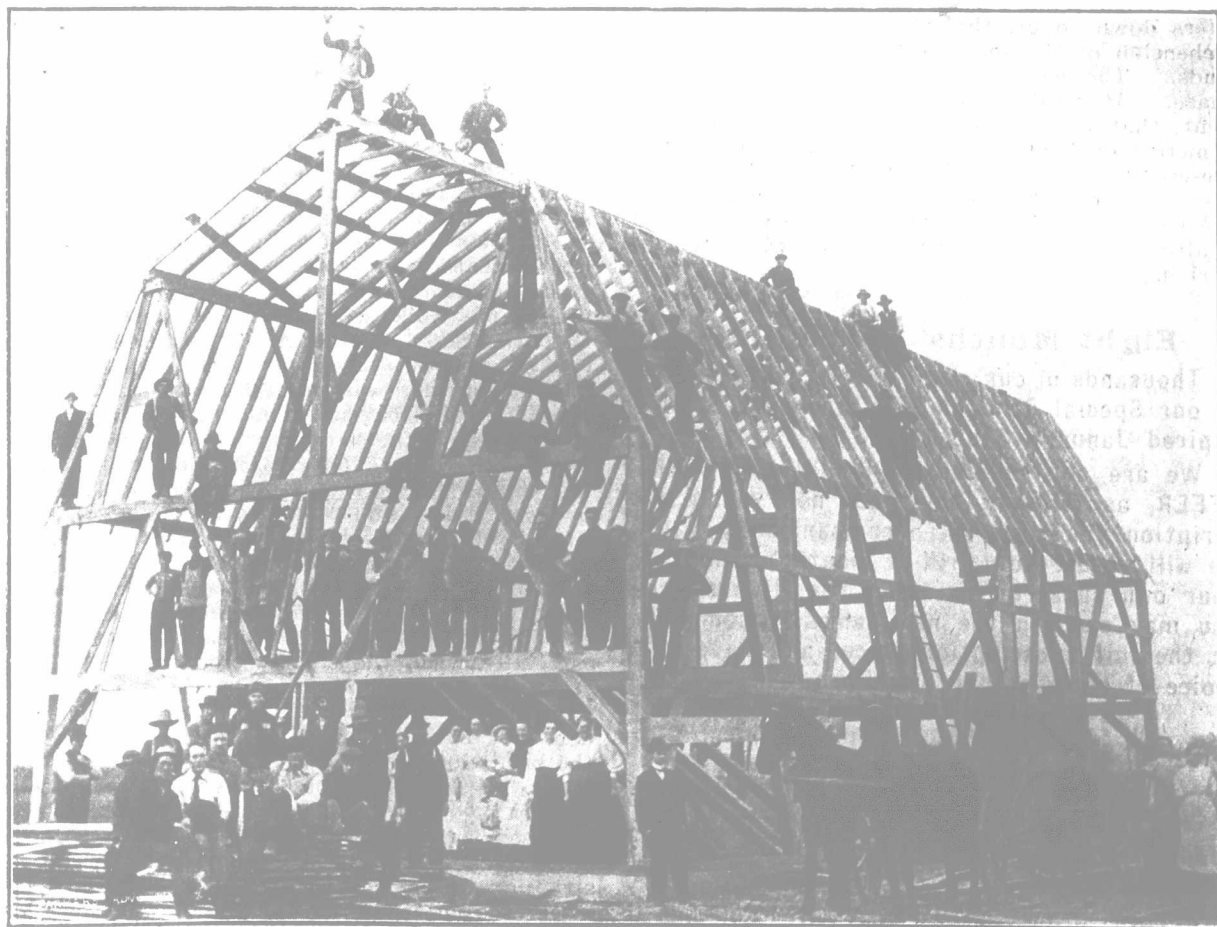
Plank frame, erected for Harmon Marr, Welland Co., Ont.
