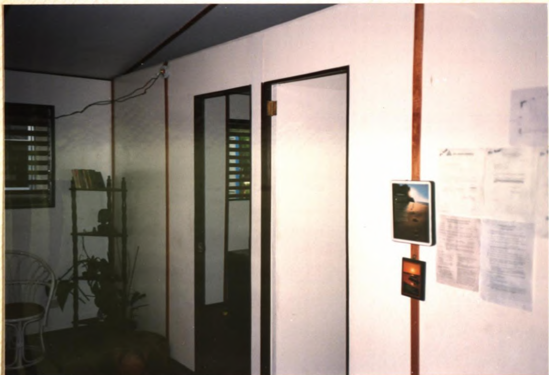
No. 32. Interior of Lukut House. 2 bedrooms on right. Note hardwood stripping on panel joints.
