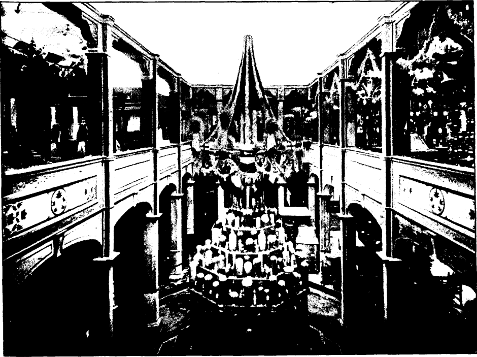
INTERIOR OF CANADIAN PAVILION—GENERAL VIEW.
