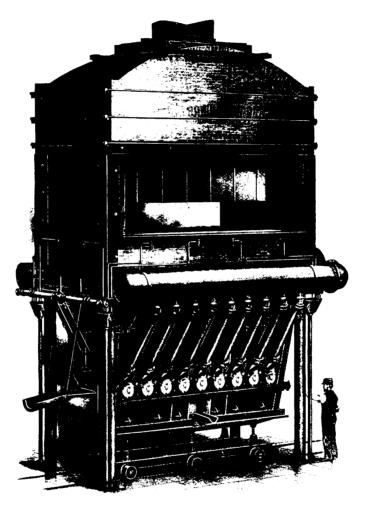
The above cut represents our latest improved type of 42 in. x 160 in. Copper Smelting Furnace, built for the Rio Tinto Copper Co., Ltd., of Huelva, Spain. The design embodies all the latest improvements recognized to be of value among metallurgists. The best material is employed in its construction, and this, together with the high-class workmanship and excellence of design, make it representative of the most complete development and advancement in Copper Smelting Machinery.
