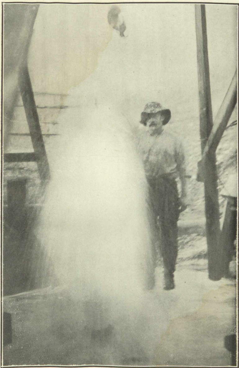
Gas Well on the Athabaska. Drilled by A. Von Hammerstein. See page 42.
