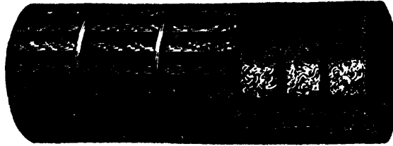
Fig. 2.—Jacket on Boiler at the Grand Opera House, New York.
