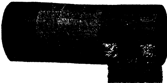
Fig. 3.—Canvas and Sheet Iron Cover Used on Boilers of the Pennsylvania Railroad Company.
