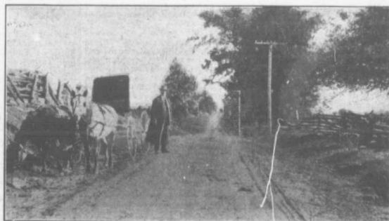
A GRAVELLED COUNTY ROAD IN HASTINGS
