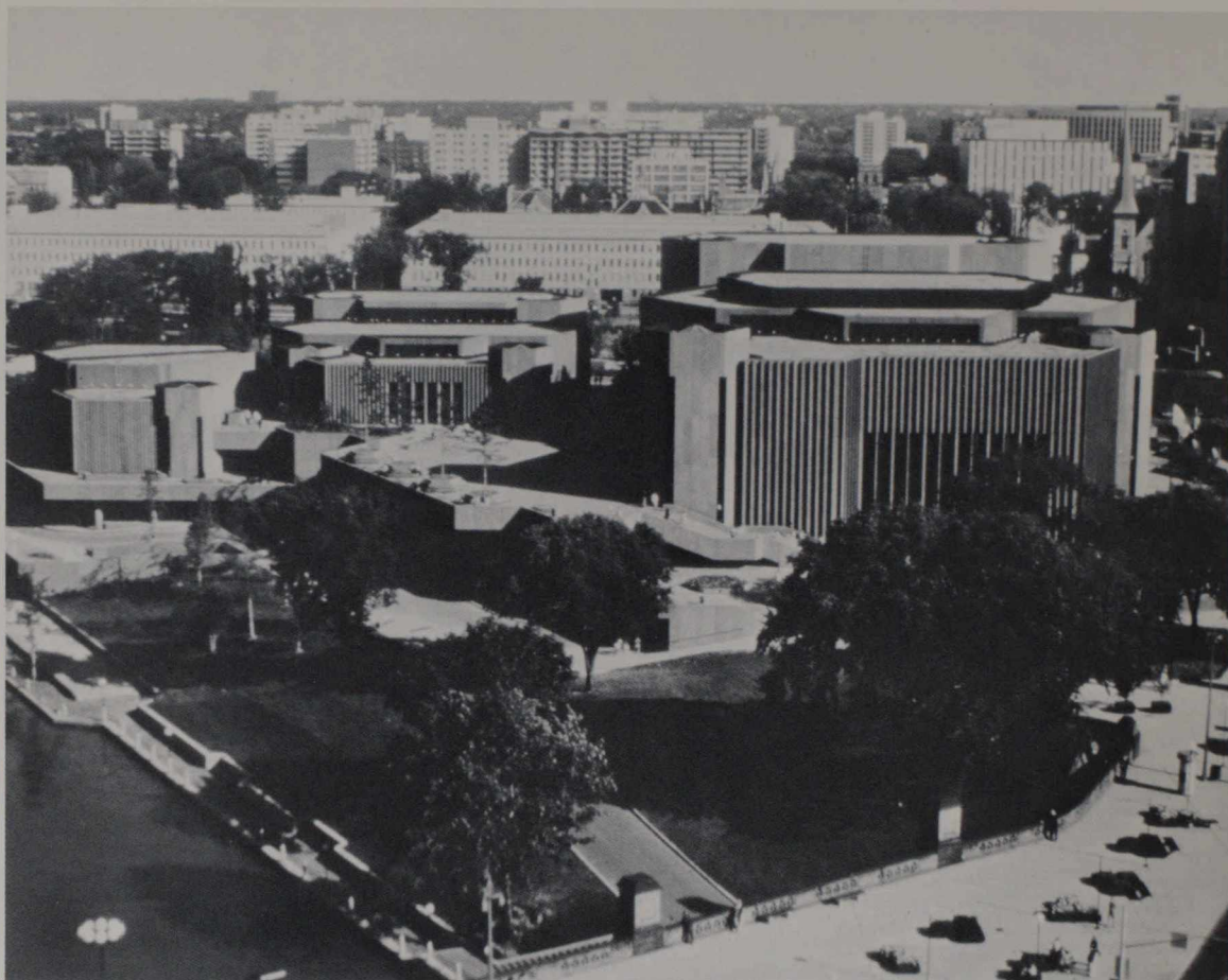
Lower center, the National Arts Centre.
