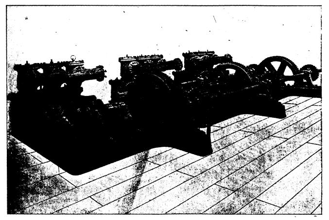
3 SETS OF GEARED THREE-THROW HORIZONTAL RAM PUMPS 9 RAMS EACH 10 INS. DIAMETER X 20 INS. STROKE.
