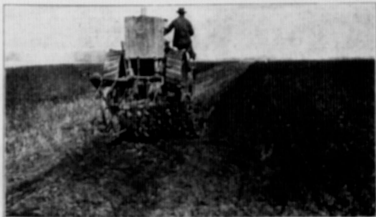
Showing the fine effect on the furrow slice by the use of the packer attachment to the plow. This is done in one operation.
