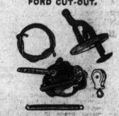
auxiliary valve, placed in the exhaust pipe. Permits exhaust gas to escape without going through the muffier. Increases the power of the motor and facilitates hill-climbing. A Muffler Cut-out is of assistance in locating engine to white and making engine troubles and making adjustments on vibrator or
