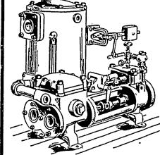
The most successful device in market for returning water of condensation from pipes and coils of steam-heating systems at the highest possible temperature to the boilers. By keeping the pipes clear for the steam it ensures a quickly operated, soiseless, regular heating service. Takes up little room. A favorite with prominent Engineers and Archi-
