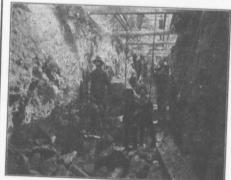
This is a view of three out of ten of our steam drills engaged in rock excavation by Messrs Laurin and Leitch, near Montreal. A full description of our Ingersoll Rock Drills, steam or air driven, is given in our Catalogue No. 81
