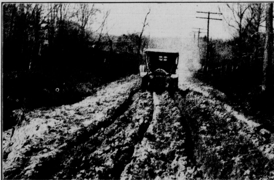
NOT ENOUGH CROWN, LACK OF ATTENTION AND CONSEQUENT HEAVY HAULING
