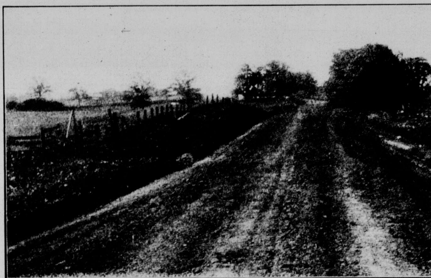
ROAD GRADED, CROWNED AND SURFACE KEPT SMOOTH BY A DRAG, CONSEQUENTLY EASY HAULAGE AND COMFORT
