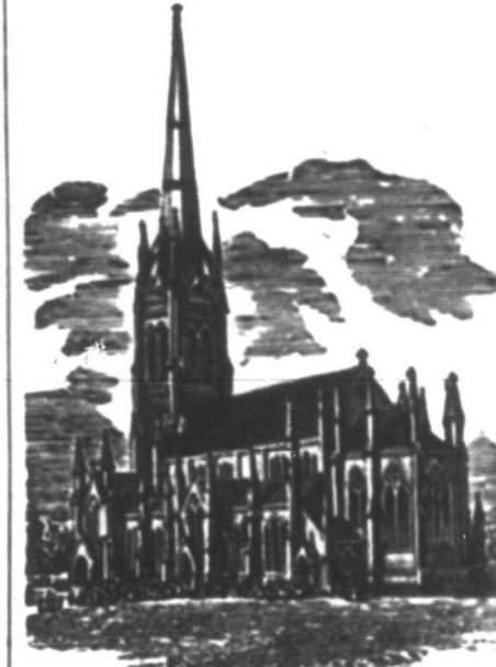
St. James' Cathedral, King St., Toronto, contains 500,000 cubic feet of space and is successfully heated with four of our Economy Heaters.
