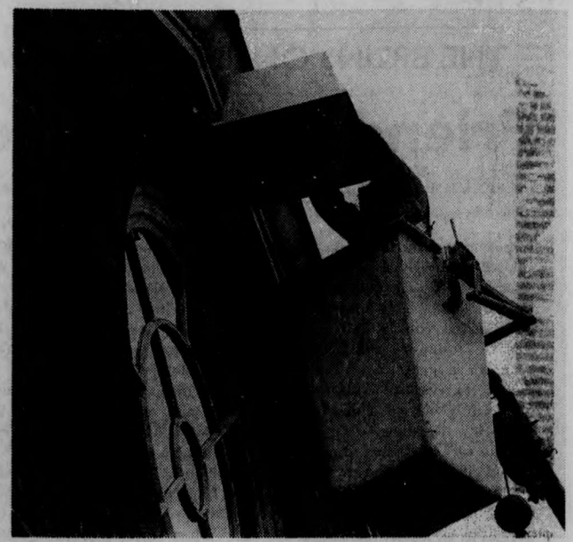
This camera was installed at the back of the Student Union Building this week, so Security can monitor campus more effectively. PAT FITPATRICK PHOTO
