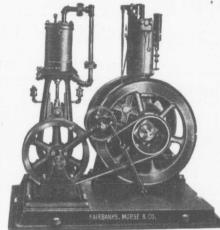
This arrangement is most convenient and economical in small sizes where the Compressor and Engine must occupy a minimum space.
