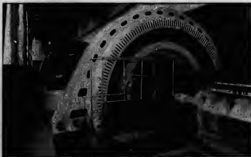
One of the 10,500 h. p. Generators (Lake Buntzen Generating Station).
