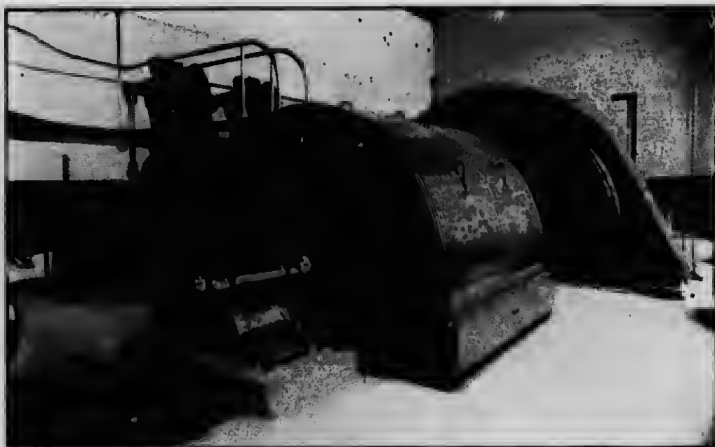
End view of one 10,500 h. p. unit, showing "Doble" wheel and governors. Lake Buntzen Generating Station.
