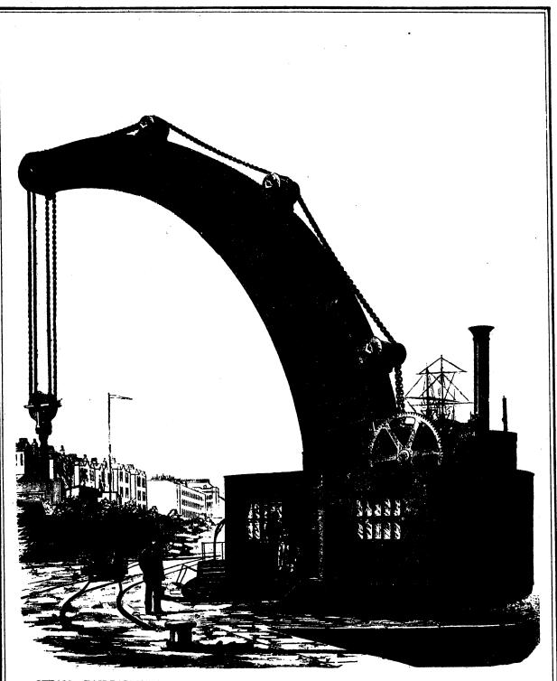
STEAM "FAIRBAIRN" CRANE, FROM A PHOTOGRAPH OF A CRANE CONSTRUCTED FOR THE BRISTOL DOCKS.
