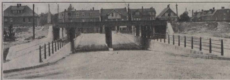
Fig. 5.—Davenport Road Subway as Completed.
