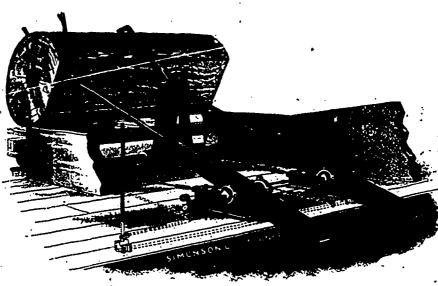
Requires no space below floor timbers. Is adapted to a mill sitting on the ground or otherwise. Does not injure the timber.
